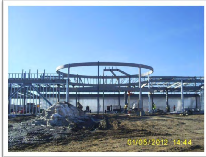
Crownpoint Court Construction (January 2012)
