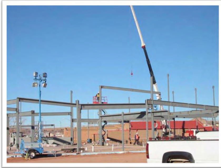
Tuba City Court Construction (January 2012)
